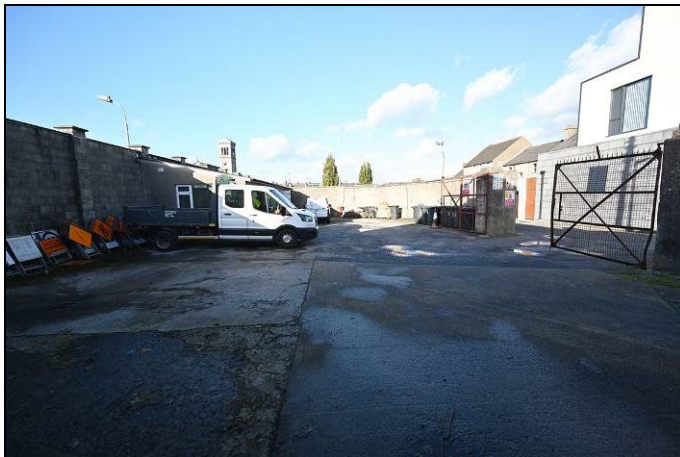
Photograph 5: Concrete surface Depot yard, looking north.
