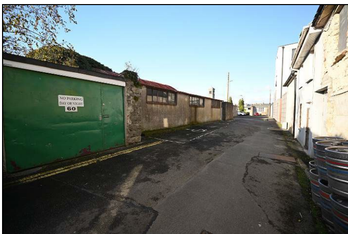
Photograph 1: TCC Depot on the west side of Stable Lane, looking northwest. The green gate marks the southeast corner of the development area. The existing boundary wall is rubble stone with concrete render as far as the splayed vehicle entrance, and concrete block thereafter.
