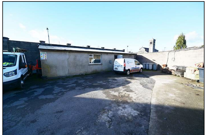
Photograph 6: Modern structure in northwest corner of Depot, to be demolished.
