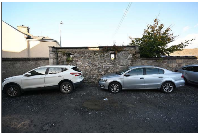
Photograph 15: View of the surviving gable-end of the structure in northern boundary wall of the parking area.
