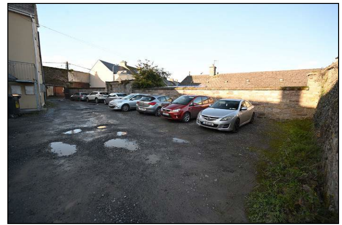
Photograph 16: View of the northern boundary wall of the parking area. The wall to the east of the gable-end is a modern stone wall, and will be retained as part of the development works.
