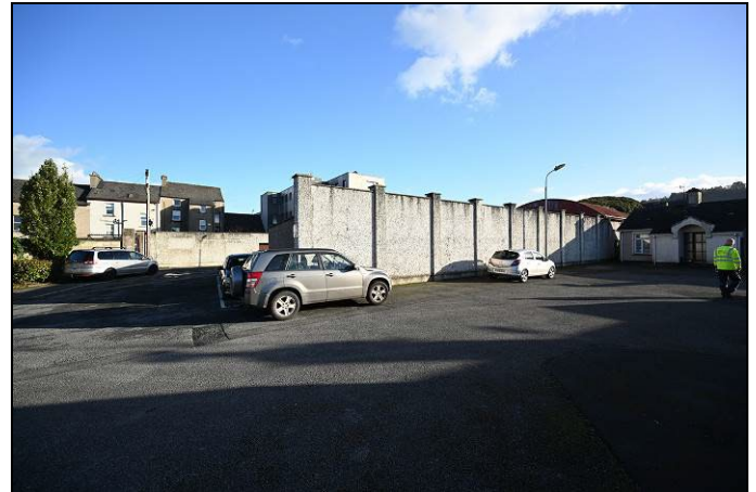
Photograph 4: Concrete block boundary along the western side of the Depot, viewed from New Lane Court, looking east.
