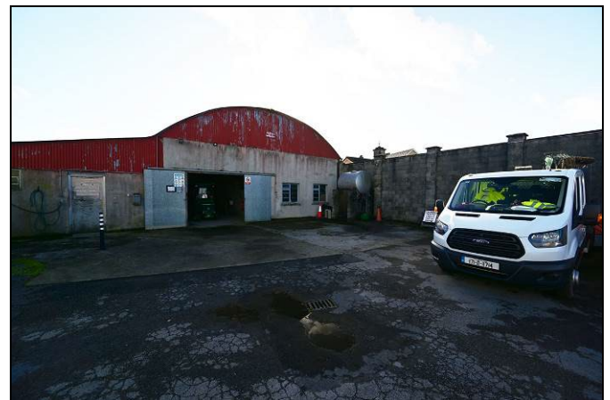
Photograph 8: Depot shed, looking south.
