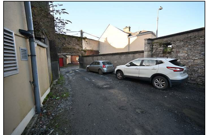
Photograph 14: View of the northern boundary wall of the parking area, easternmost section. This concrete block rendered wall will be removed. To the right of it the stone fabric, with window apertures, appears to be the surviving gable-end of another structure shown on the mid-19 th Century Valuation map, see Figure 14 above.
