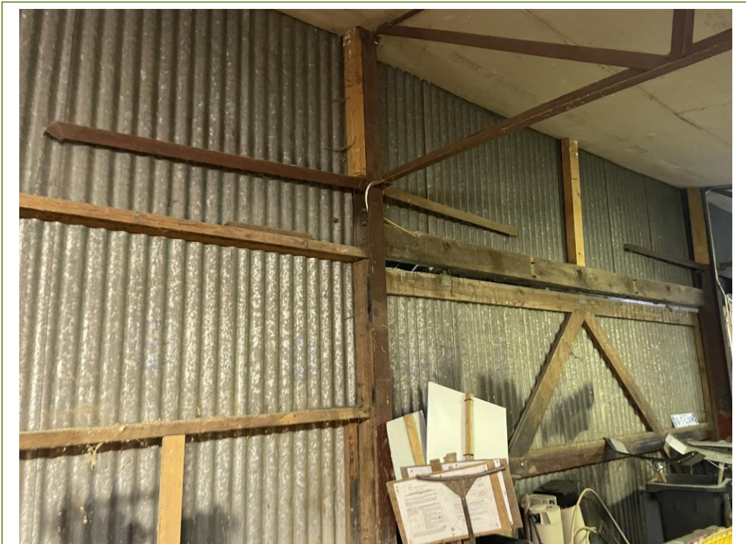
Wall cladding in the store building
