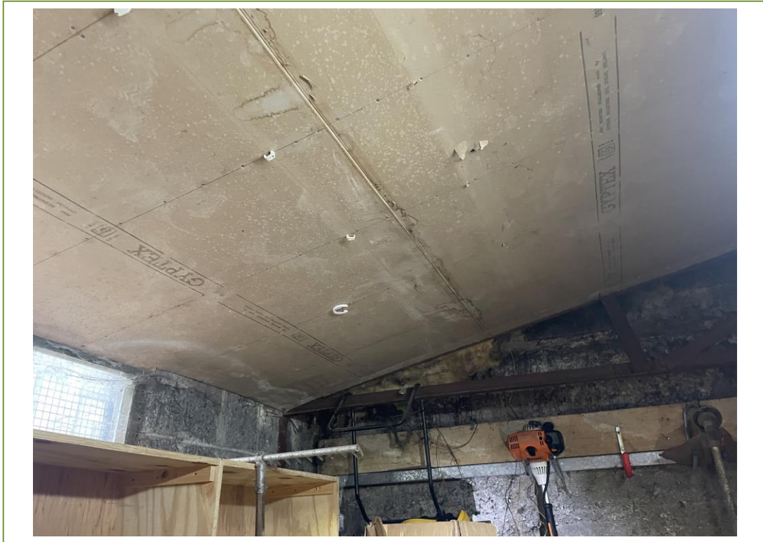
Plasterboard ceiling boards
