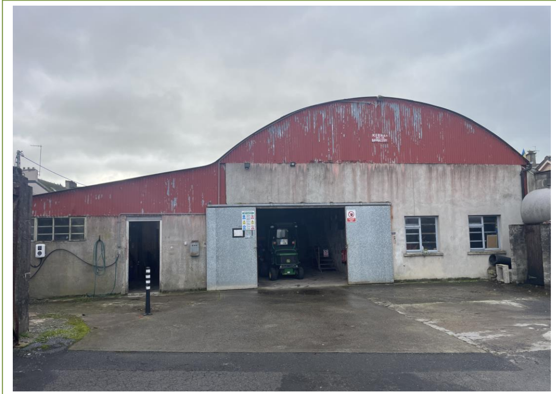
Roof cladding in the store building
