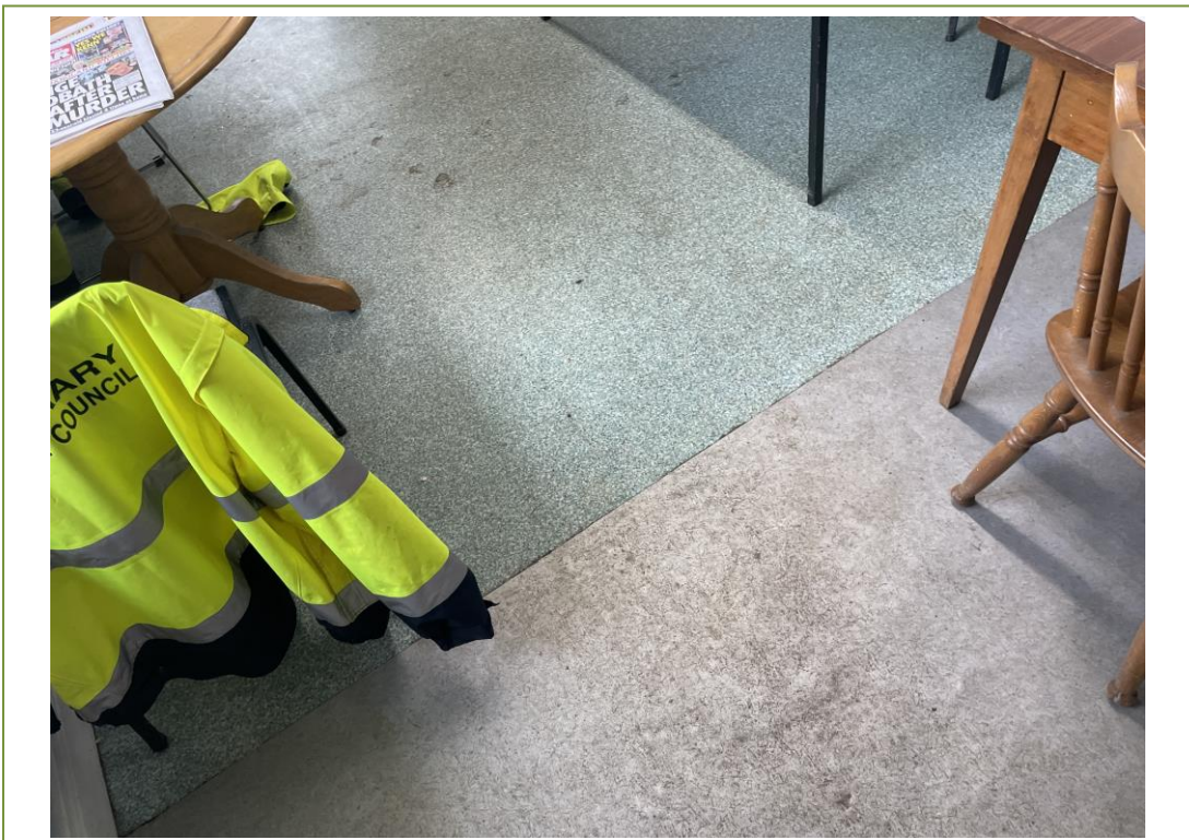
Floor covering in the canteen
