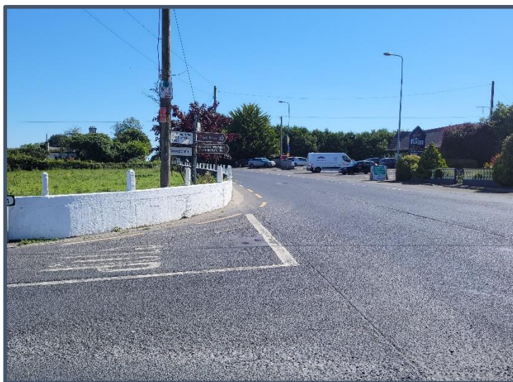
Figure 3.3 Poor visibility at entry from L4131
