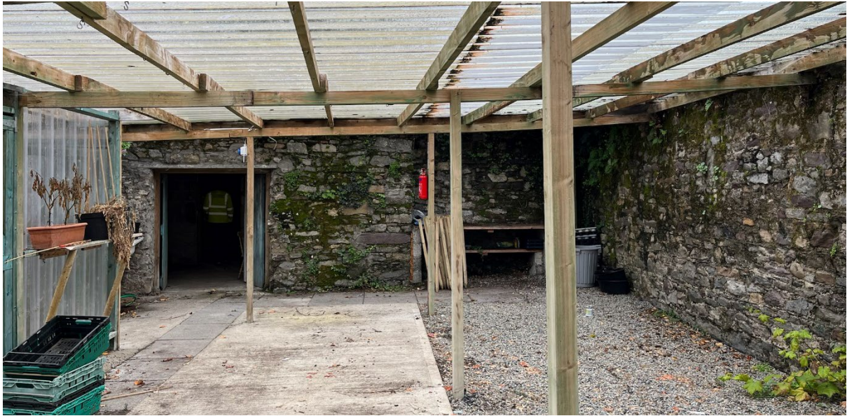
Figure 13: Covered yard at centre of site - view towards east
