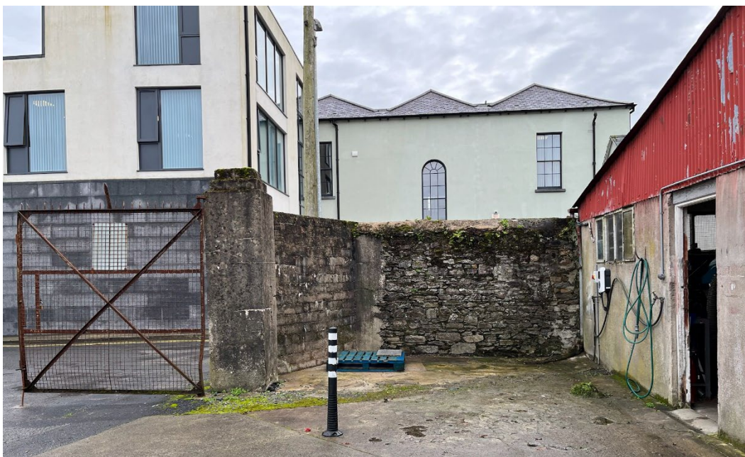
Figure 8: Site boundary wall on eastern side, taken from within site
