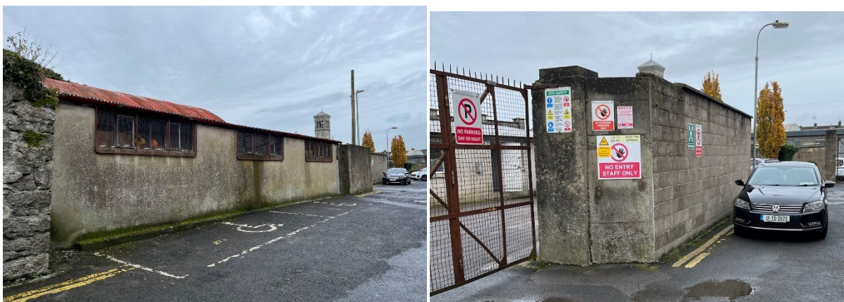
Figure 6: Eastern boundary of site, showing single-storey shed to be demolished (left) and view of wall towards north of Stable Lane (right)
