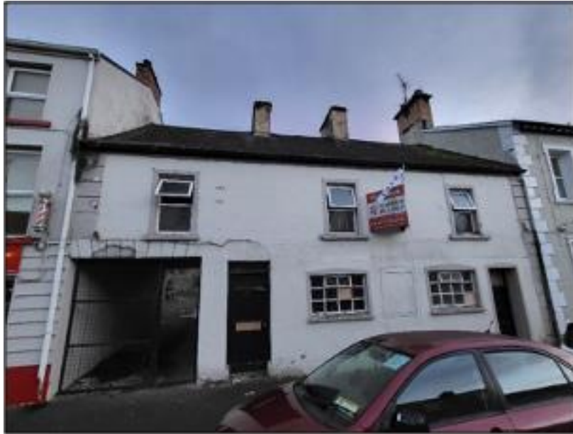
Frontage of building under survey on Main Street Ballinamore
