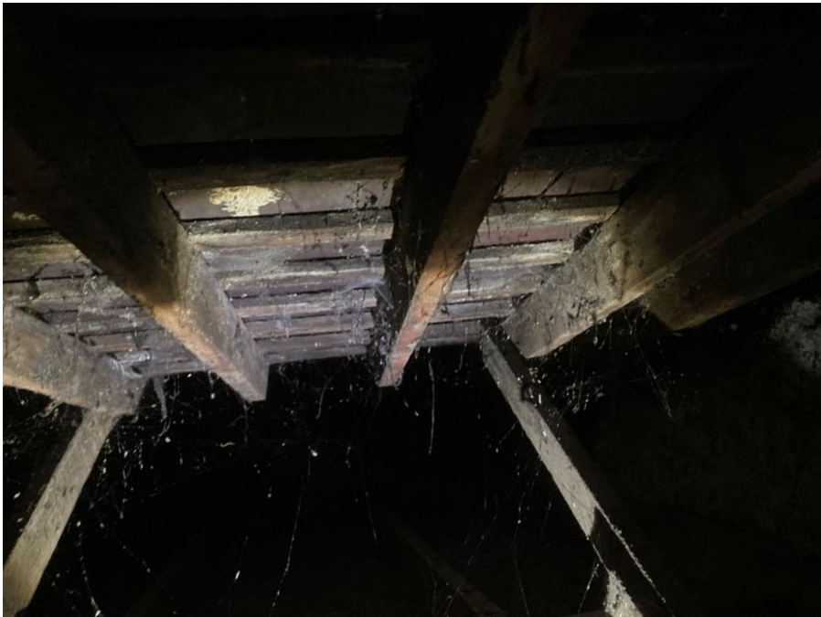
Fig. 4. A view of roof underside showing cobwebs.
