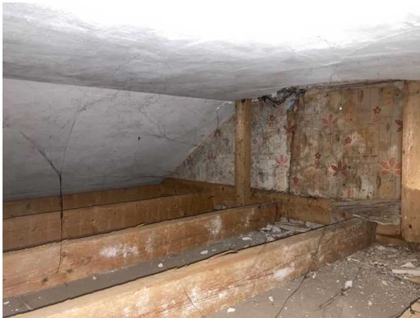
Fig. 2. Area within suspended ceiling over one of the first floor bedrooms.
