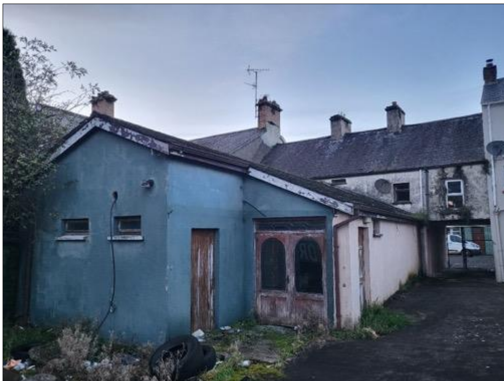
Figure 2. View of the rear of the property.
