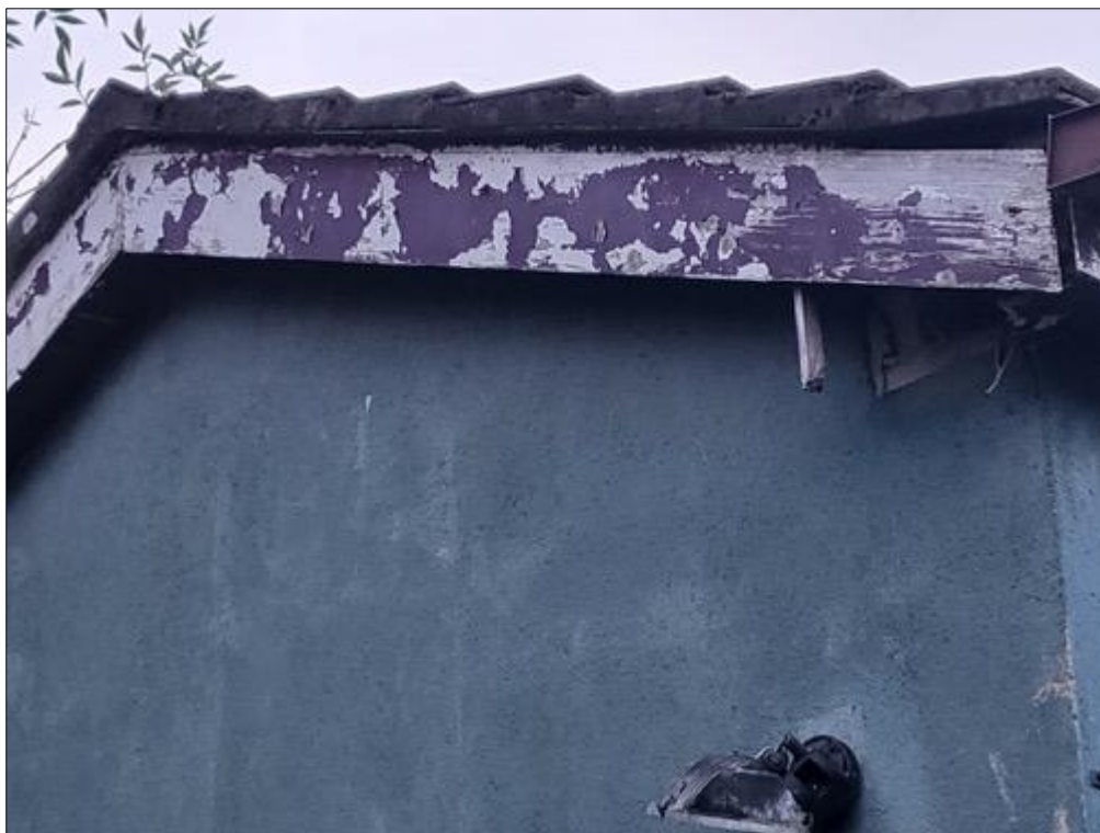
Figure 4. Fascia along the rear extension gable.
