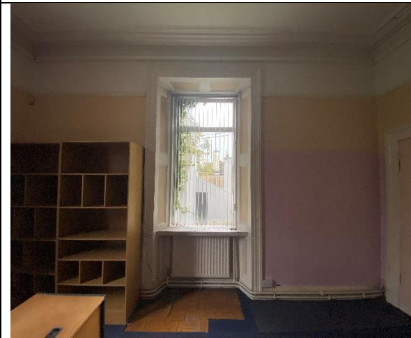
West facing view (Room 8) panelled window surround, skirting, cornice, Panelled door.
