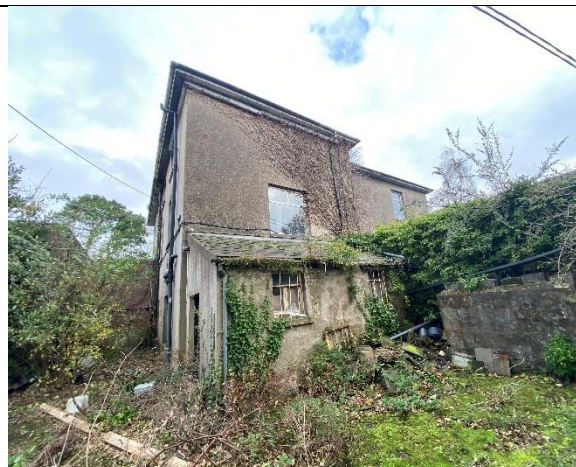
Rear (west) facing elevation. Note lean to and dividing (likely later) wall.
