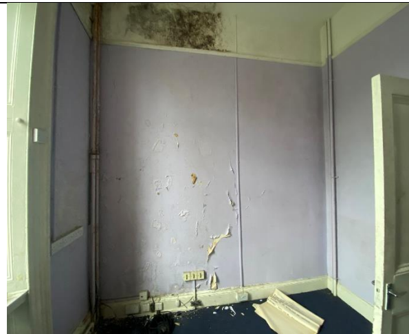
Room 9, ground floor, proposed area for installation of lift. New partition proposed and removal of skirting and alteration to floor
