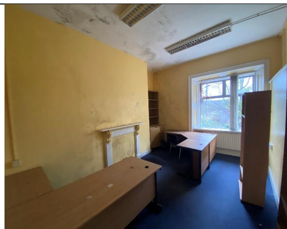
Ground floor (Room 10) facing west elevation (Rear). Original fireplace and panelled window surround. No cornice.
