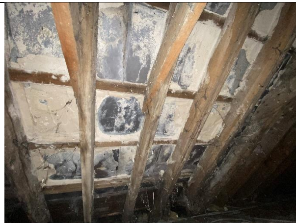
Example of surviving lime parging on internal pitch of roof.
