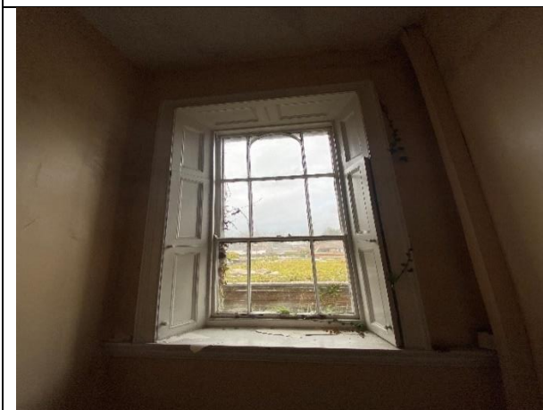
Tripartite timber sliding sash window to half landing between ground and first floor.
