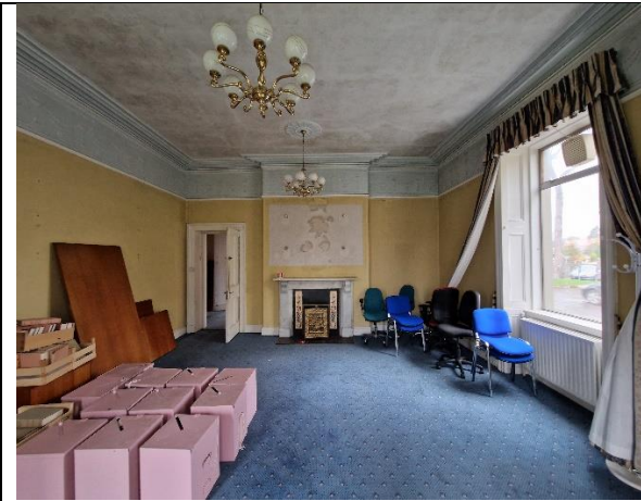
Ground floor (Room 7) Original fireplace, Cornice, ceiling rose, skirting, architrave, panelled door, window surround and box.
