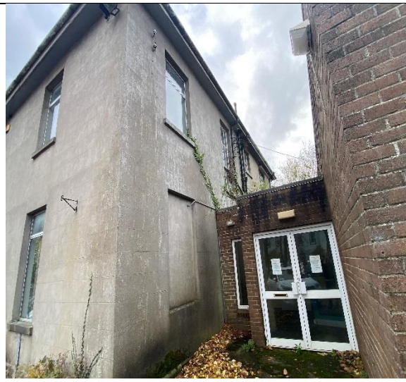
Side (north) facing elevation with join of existing modern library building and Dan Breen House. Note blind window.
