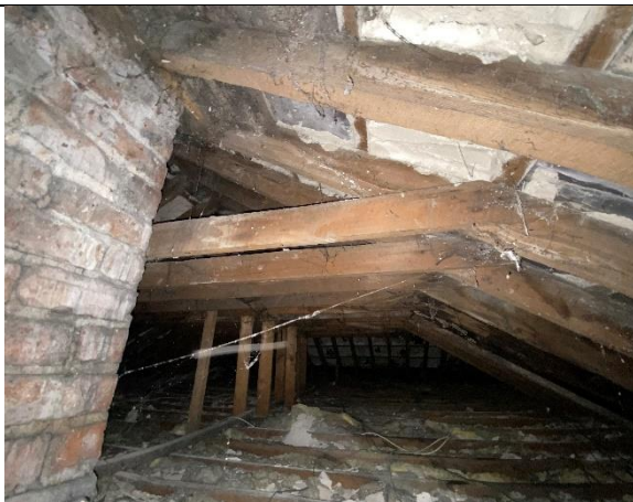
Detail of collar tied roof construction
