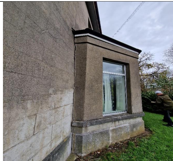
Destabilized bay window to south elevation. Note cracking to joint.
