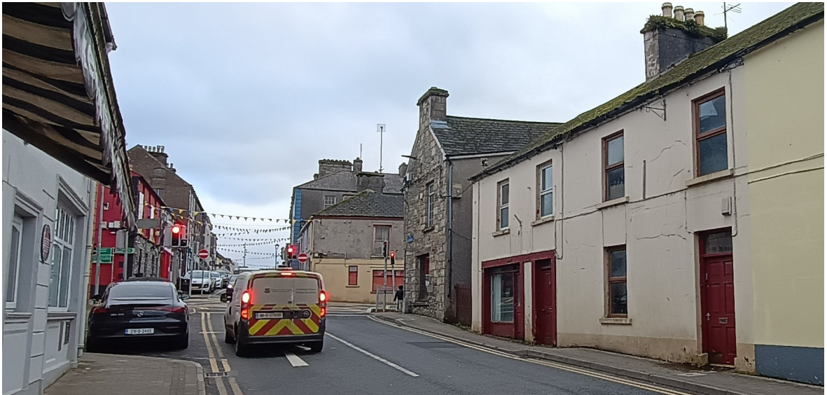
Plate 2.1 – R280 Sean Mac Diarmada Street, Manorhamilton – Looking south with the proposed development site on the right
