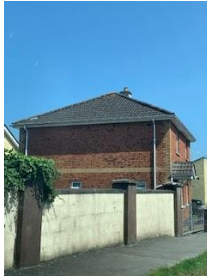
Figure 2: View of facade and elevation to be extended
