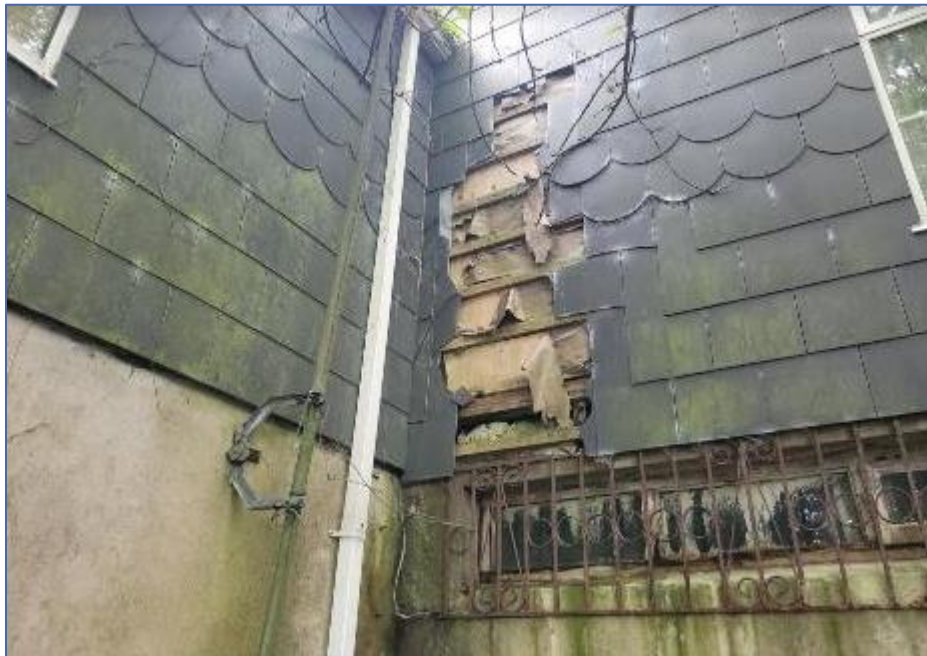
Asbestos Roof Slates to rear – Poor condition
