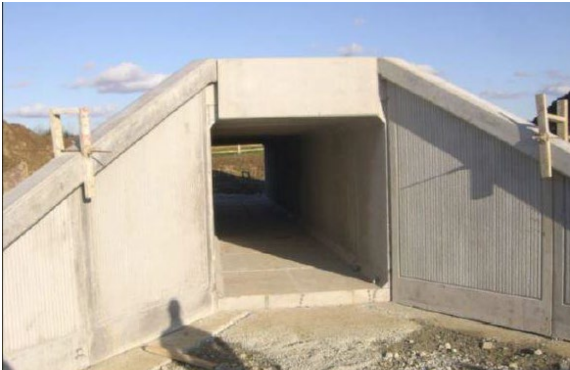
Figure 1: An example of a typical pedestrian road underpass (pre-cast construction).
