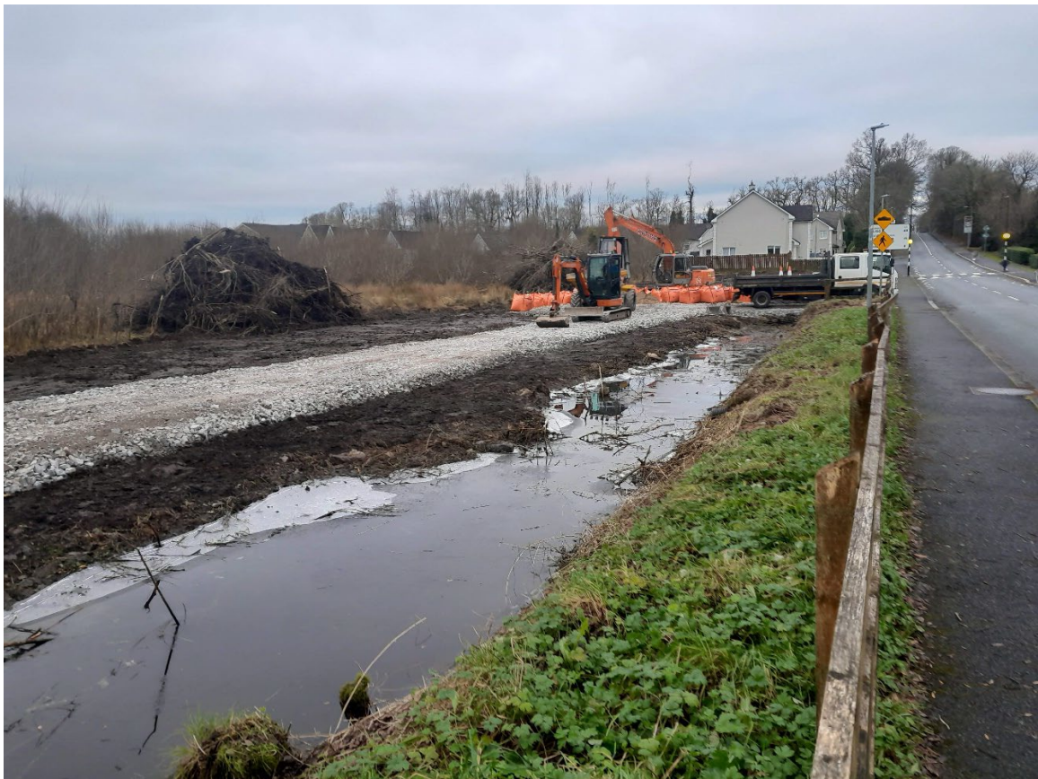
Fig. 3: Image of emergency temporary works undertaken in January 2024
