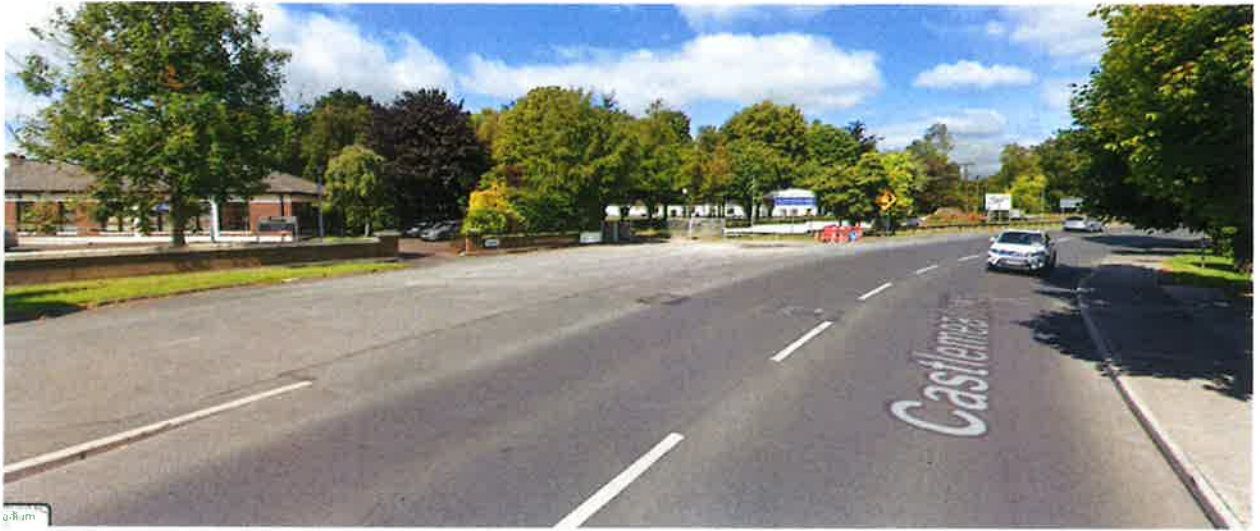
Photo of the Wide entrance outside Coláiste Mhuire with no defined path for pedestrians or cyclists
