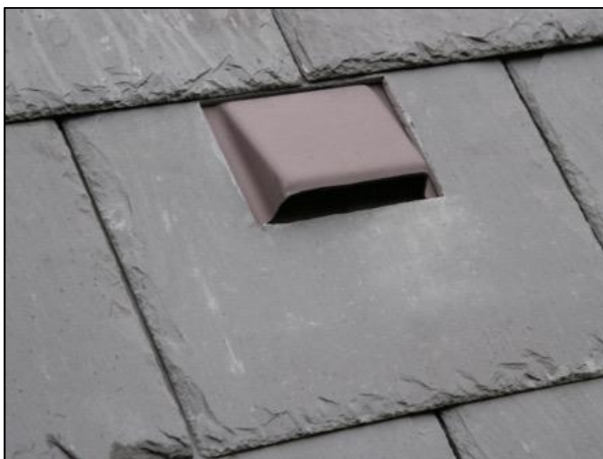
Figure 7. Example of an adapted roof slate that permits bat access to a roof space.
