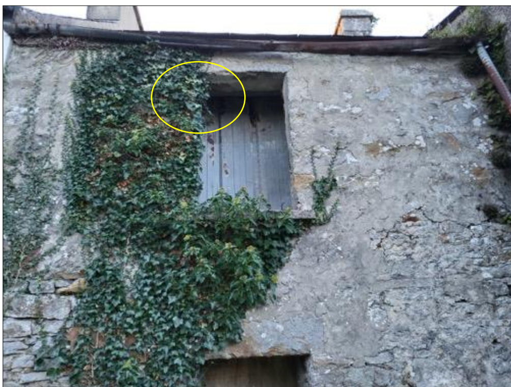
Figure 7. Second storey rear window from which a single soprano pipistrelle emerged.
