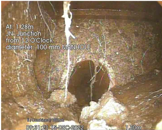
MH2 TO UPS5_1-30m_093121.jpg, 00:00:10, 1.30 m Junction at 12 o'clock, 100mm dia, MANHOLE
